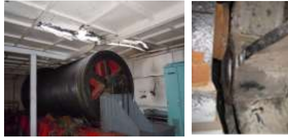
Fig.1 Drum Shaft of Lifting Mechanism of Crane
